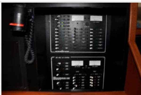
AC and DC control panels
