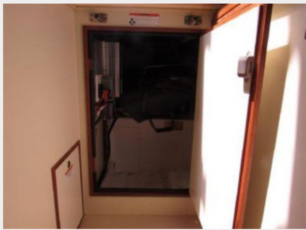
Engine Access Under Companionway
