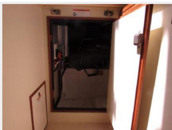
Engine Access Under Companionway
