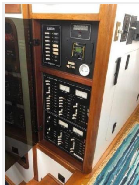
Electric Panels at Companionway
