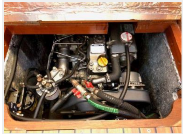
Yanmar engine with access fwd and aft ends
