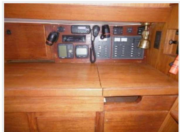
Nav and Electrical panel
