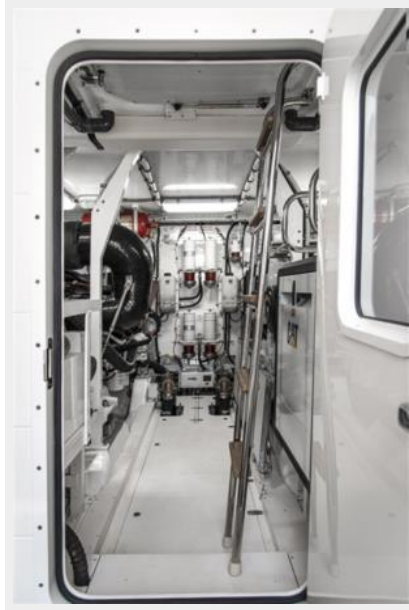
Engine room door
