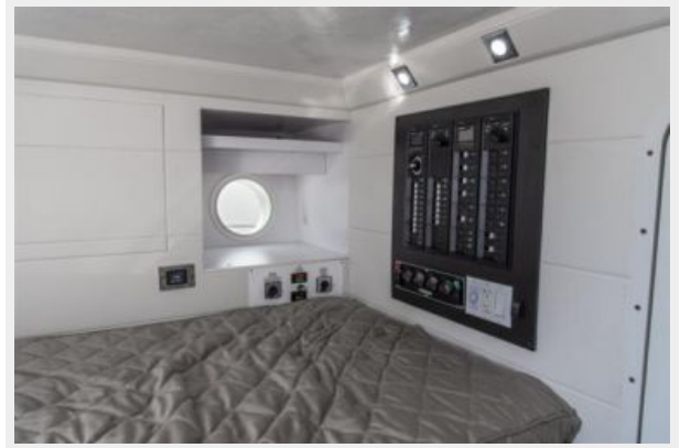
Crew area electric
