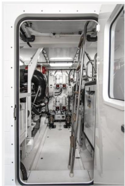
Engine room door
