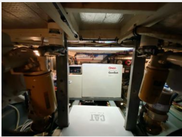
engine room looking forward
