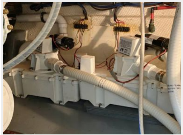
2019 New Vacuflush heads and plumbing
