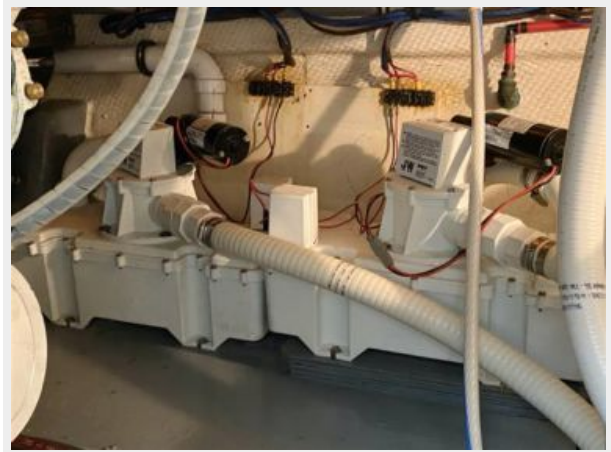
2019 New Vacuflush heads and plumbing
