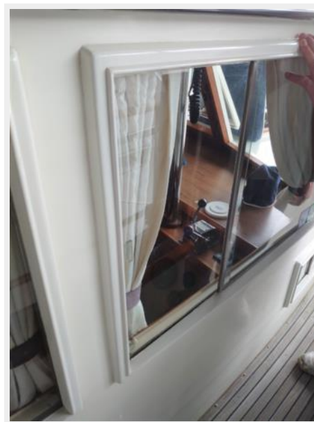
Exterior window frames
