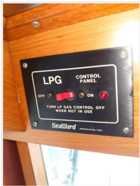
LPG Control Panel over head at Lower Helm
