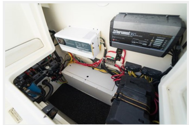
2016 32 World Cat Engine Room
