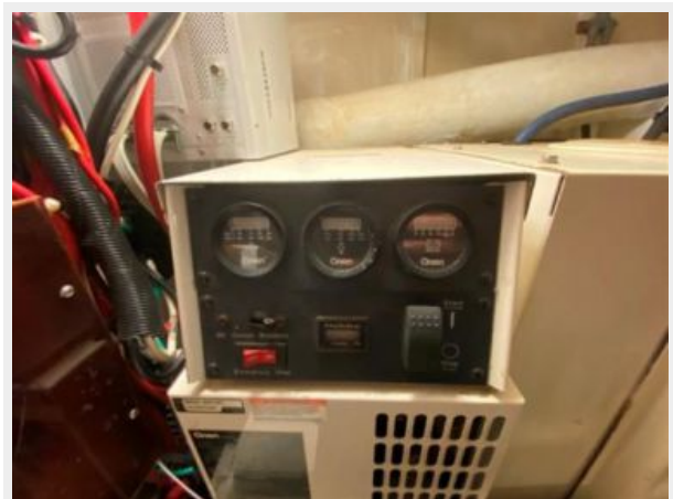
331 Generator Control Panel
