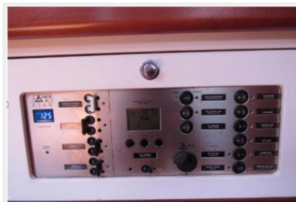
DC electrical panel
