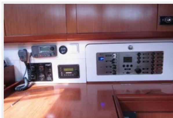
DC Electrical panel and instruments at nav station
