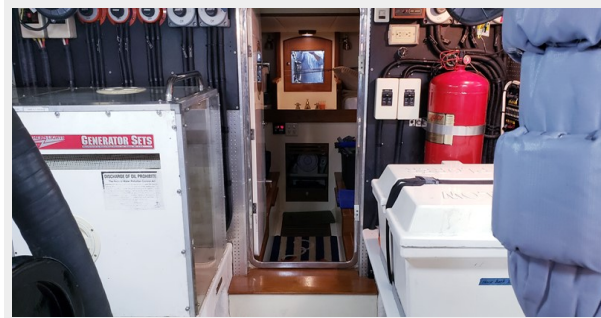
Engine Room Looking Aft into Crew Quarters
