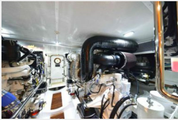
Engine Room facing Starboard
