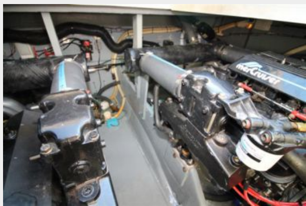
Engine room looking aft
