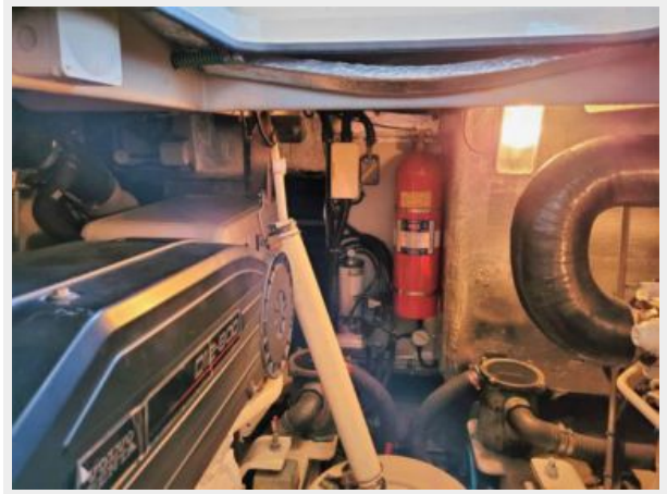
Engine Room Aft to Stbd
