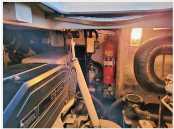
Engine Room Aft to Stbd
