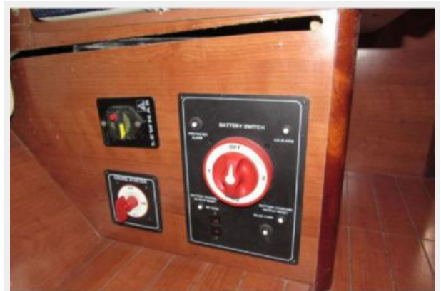
Battery switches & windlass breaker
