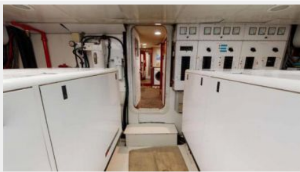
Engine Room Looking Forward
