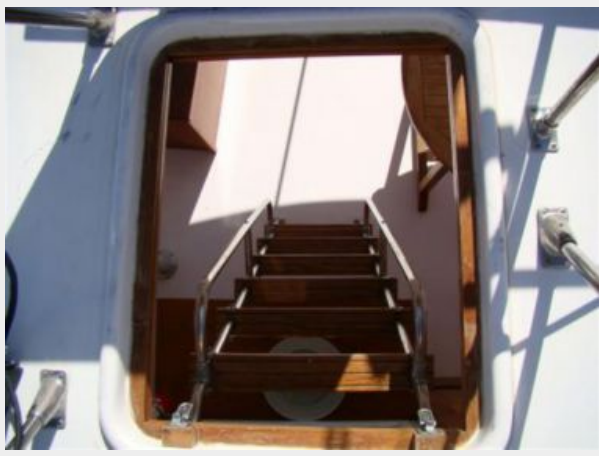
32. Fly Bridge Stairs
