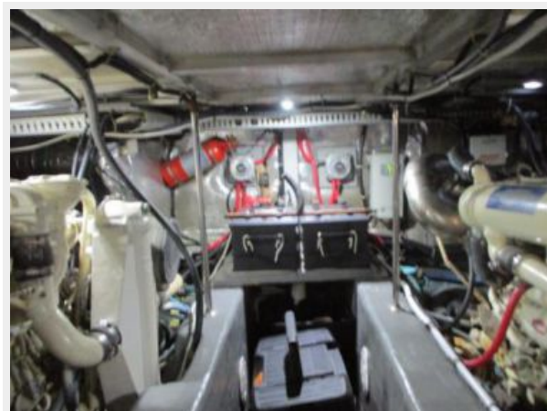
57. Carver 500 Engine Room Aft
