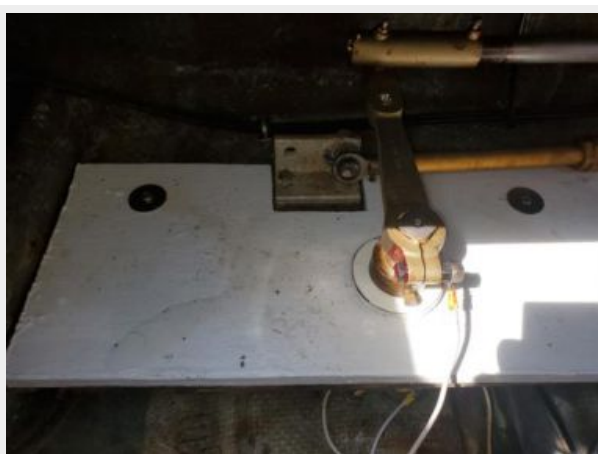
New rudder bearing and support table (starboard)
