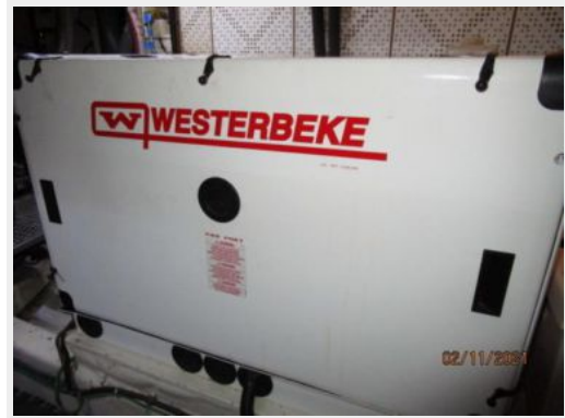
69_2777975_49_defever_generator_sound_box
