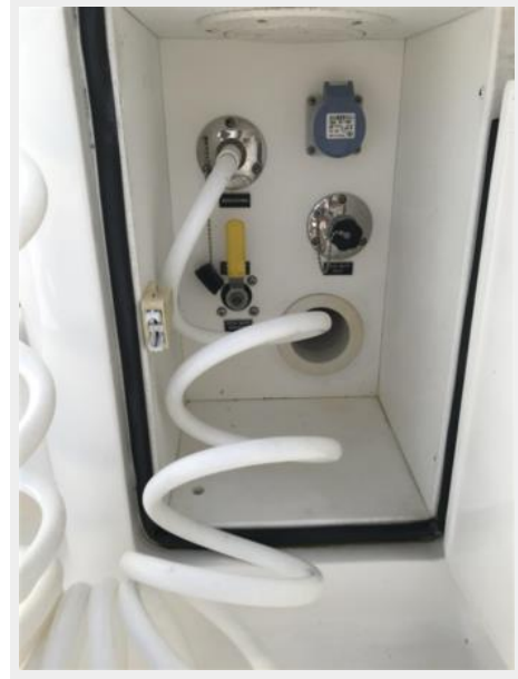
wash down/utility cabinet
