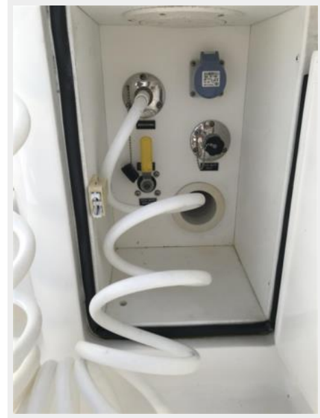
wash down/utility cabinet
