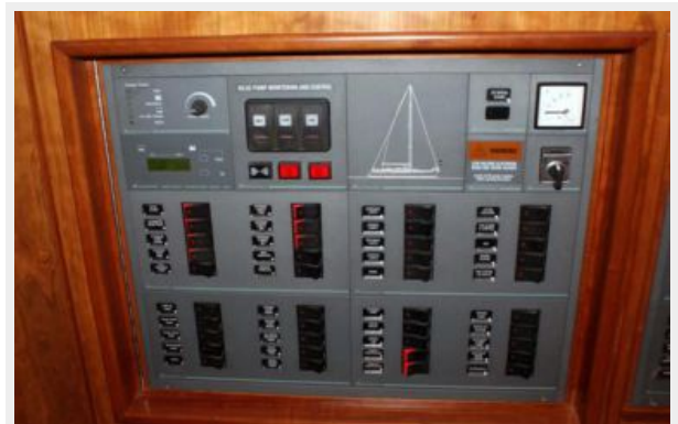
Main DC Panel
