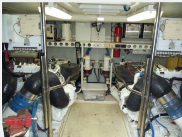
Engine Room Looking Forward
