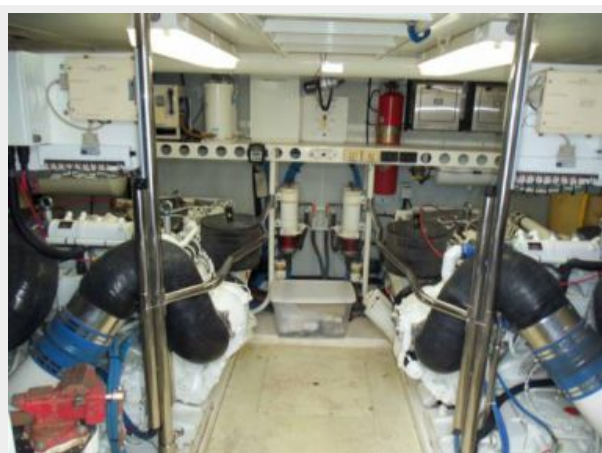
Engine Room Looking Forward
