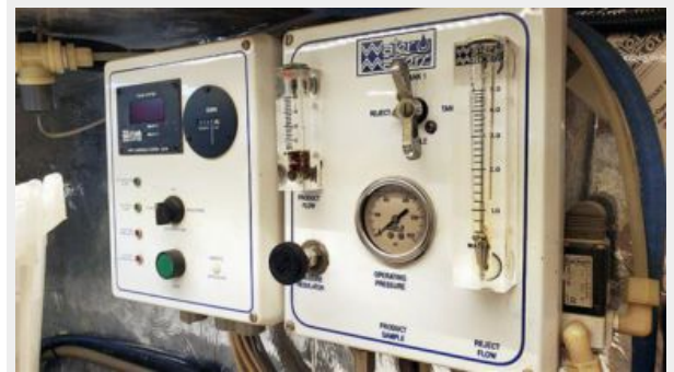
50MECHWaterMakerControlPanel
