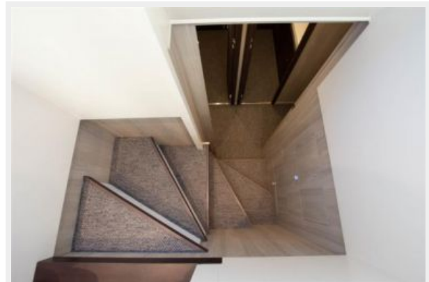
Access to crew area
