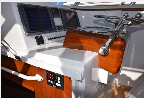
Cockpit A/C control panel in reach from helm
