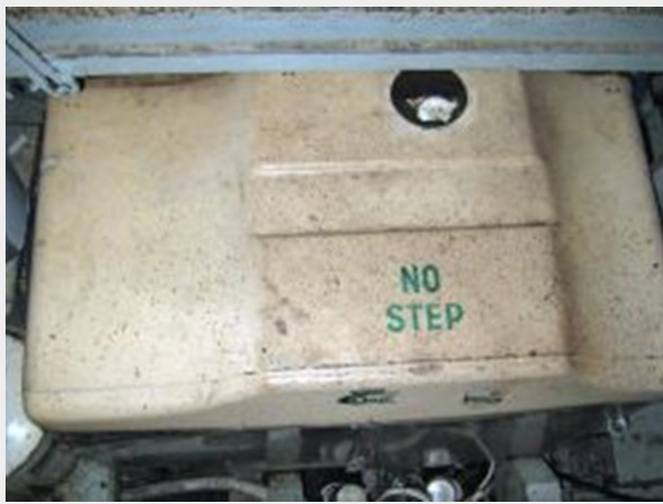
Generator with sound shield
