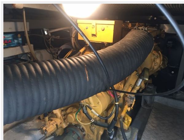
Azimut 36 Fly - Motor Yacht - interior - Engines Room - IMG_1697
