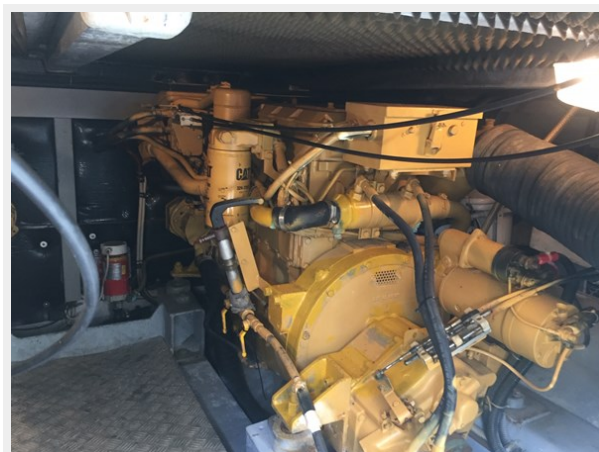
Azimut 36 Fly - Motor Yacht - interior - Engines Room - IMG_1698
