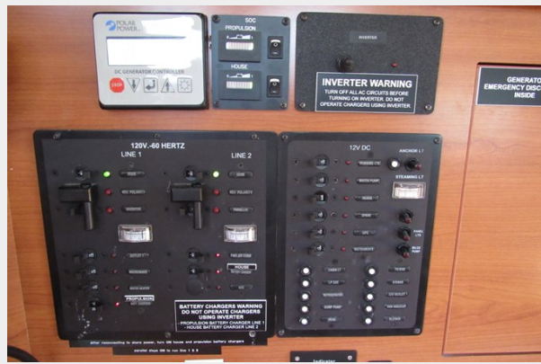
Electrical panel, regulator etc
