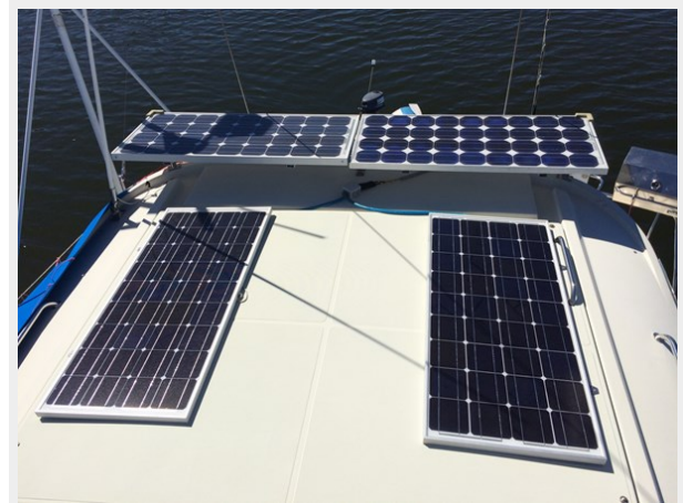
Solar panel array
