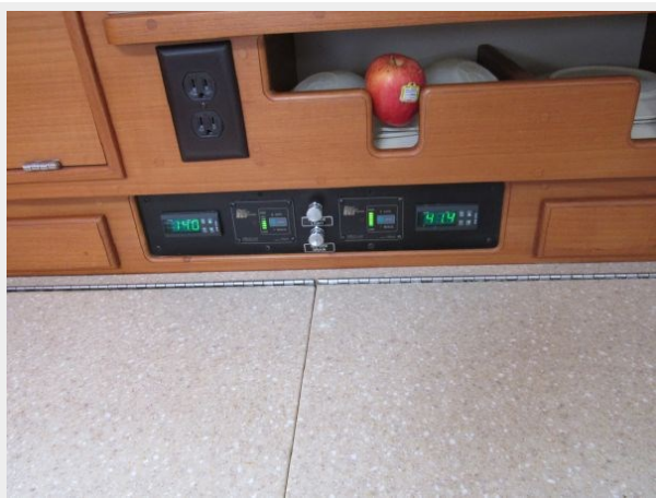
Digital refrigeration controls
