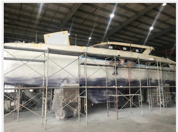
OC50 final finishing
