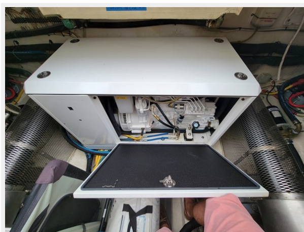
New Northern Lights Generator
