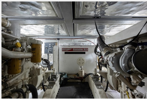
We're Comin'_Engine Room4
