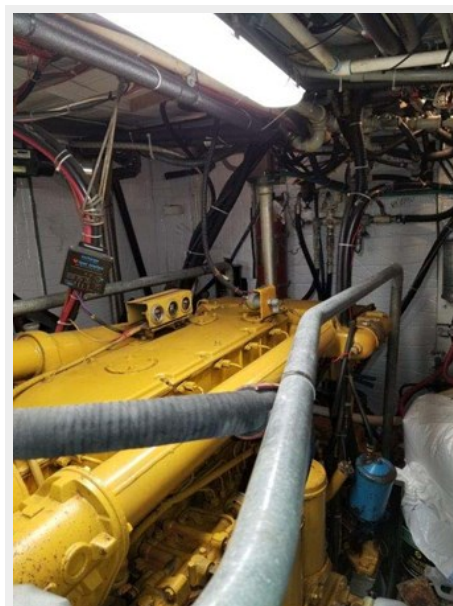
Starboard Side Main Engine
