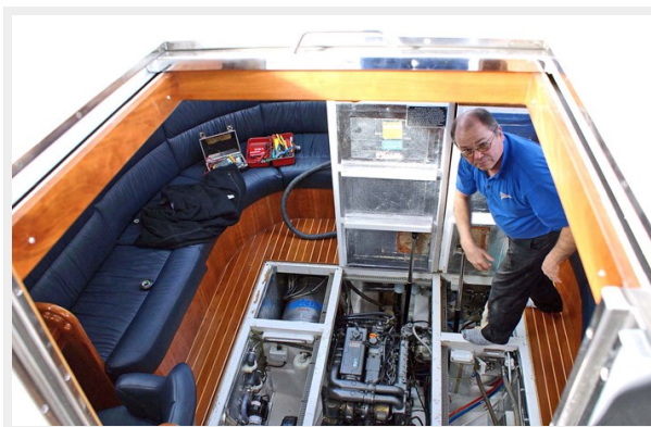
Main Salon Engine Access
