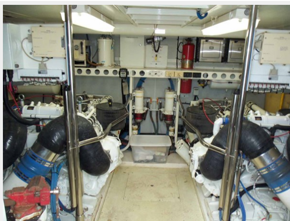
Engine Room Looking Forward
