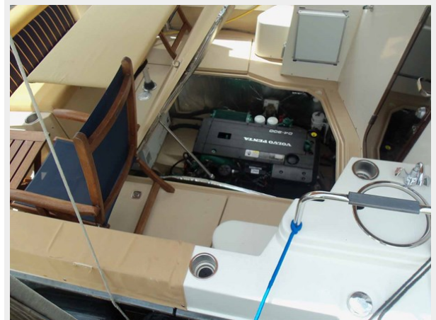
Engine Room Access
