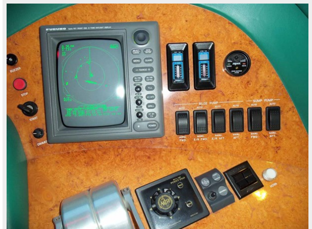
Helm Detail to Starboard
