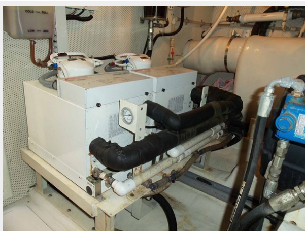
Chilled Water AC
