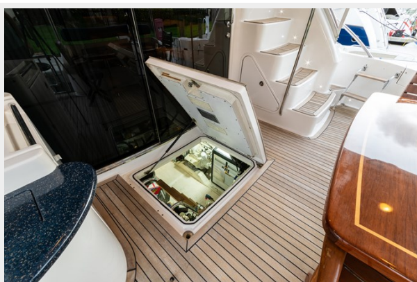
Engine Room Entrance
