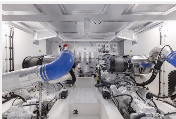
M 70 Engine Room
