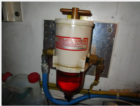
68_2780622_45_symbol_generator_racor_fuel_filter
